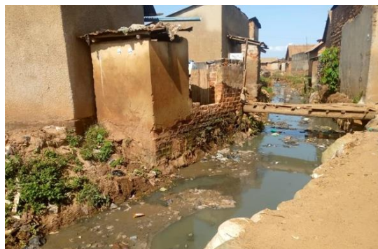
Poor sanitation and flooding, Kampala informal settlements, in, Gotto, 2022
